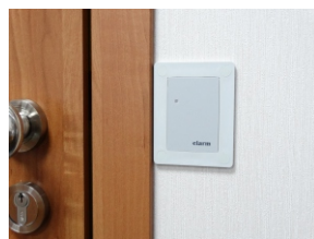
GS-280 installation under plaster
