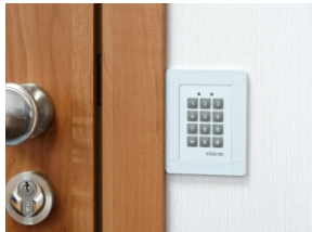
GS-280K installation under plaster
